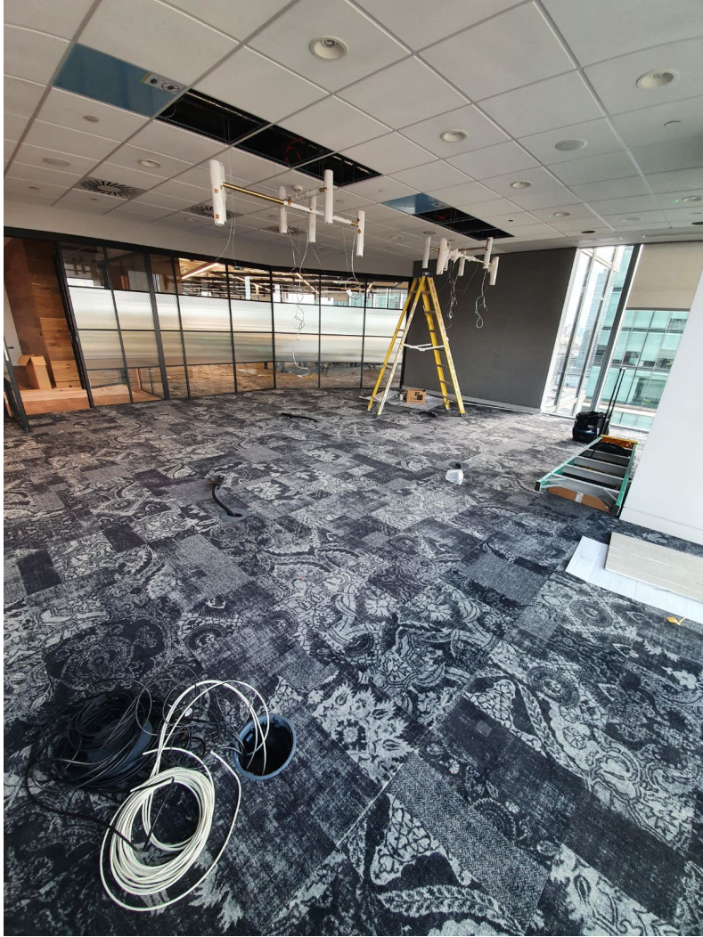
PERIMETER LOOP INSTALL
